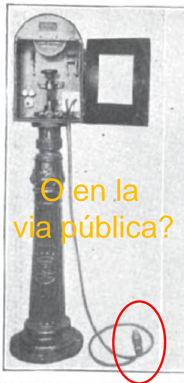
FIGS. 1 AND 2—CURB CHARGING STATION FOR ELECTRIC AUTOMOBILES
